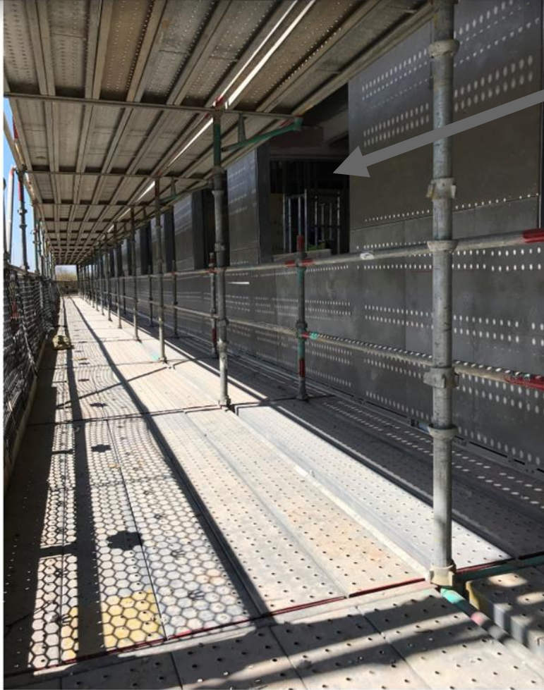
Above: Gridline E/1-9 First Floor SFS and CP board installed
