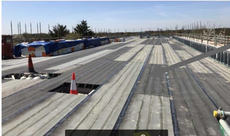
Above: Site Eye view 1500hrs Friday 23 rd April 2021 Below: Roof VCL installed and Insulation delivered
